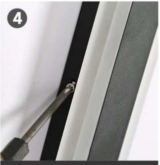
Tighten the removed screws to the plate, the installation is complete
