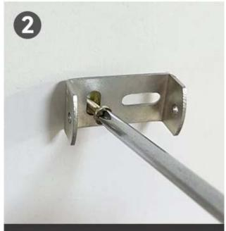
Install the hanging plate on the wall, punch holes, and fix it with screws
